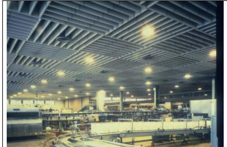
Figure 1: Sound absorbing baffles in a bottling plant
